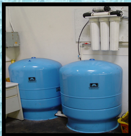
Typical Allied R/O System Installation
